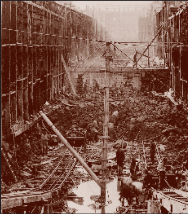
Following the purchase of the locks by the Corps of Engineers, a major renovation was undertaken. The lock chambers were deepened from 3 feet to 6 feet as a response to the increased need for passage by deeper draft vessels.
