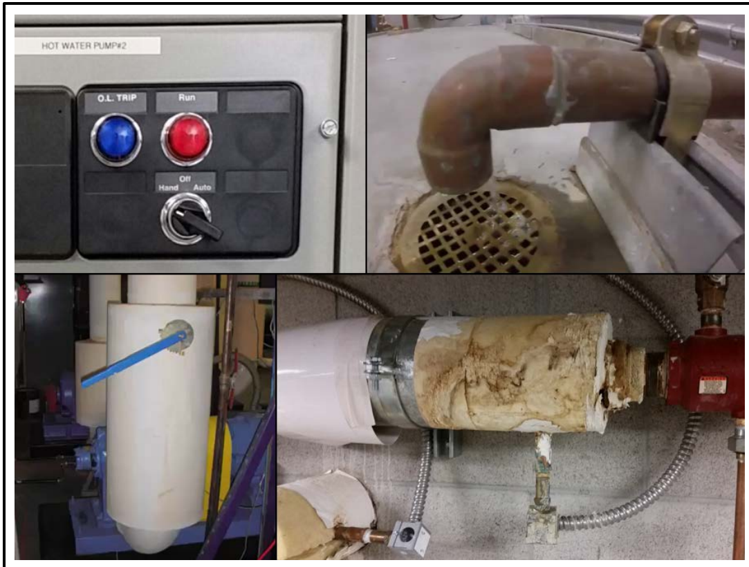
Figure 13. Examples of obvious indicators of performance: an Hand-Off-Auto (HOA) switch in hand mode may be accidental or indicative of a greater problem (top-left); active condensate drain may indicate unnecessary cooling (top-right); throttled pump discharge valve could mean oversized equipment (bottom-left); improperly installed sensors may be misleading control systems (bottom-right).
