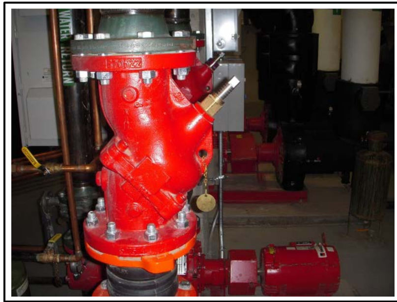
Figure 19. Pump discharge valves offer clues into oversized equipment opportunities.
