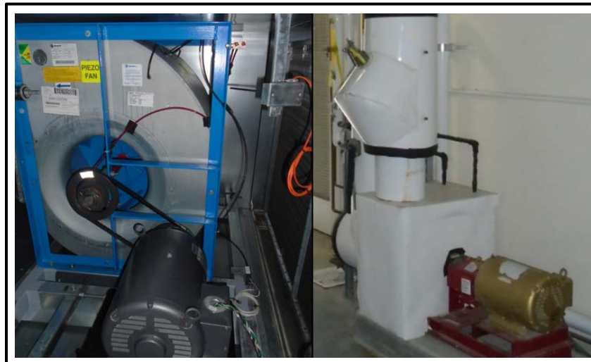
Figure 21. Most fan and pump motor systems can be readily retrofit for VFD applications.
